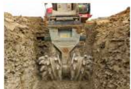
Trenching & Pipeline construction
